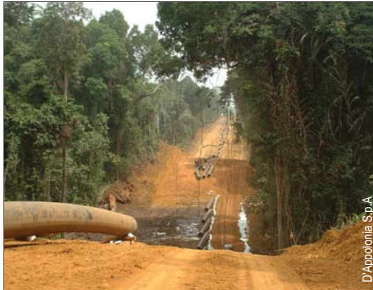
Pipeline stringing in the rainforest of Cameroon.
