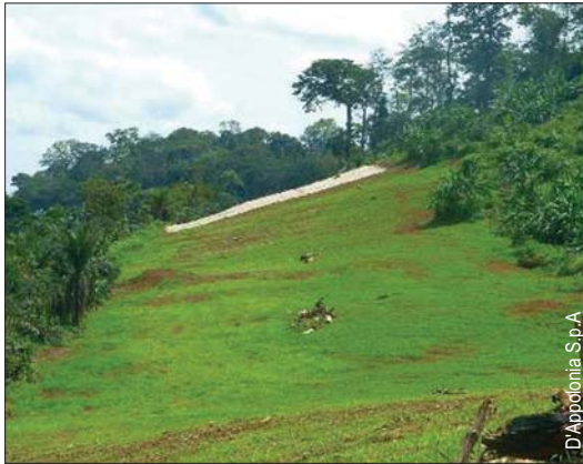
Completed restoration along the pipeline route.
