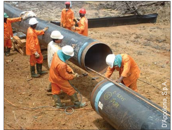
Preparation for pipeline welding.
