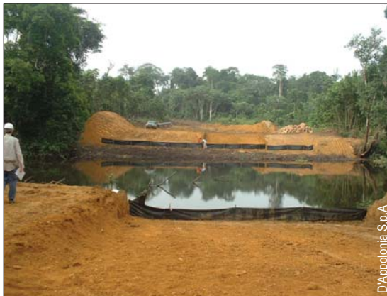
Erosion control measures on a river crossing in Cameroon.
