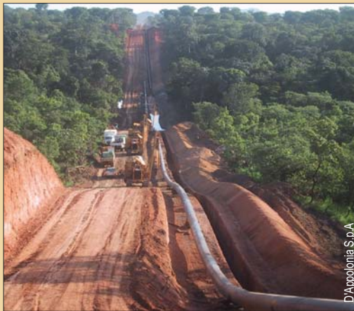
Pipeline trenching in Cameroon.
